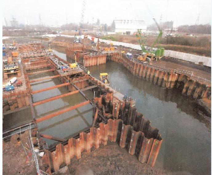
This allowed immediate commencement of production anchors using working loads of up to 1100 kN and acceptance test loads of 1650 kN. The £600k contract should achieve early completion by Christmas 2007.
