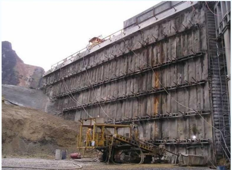
Photo 1 Freeport Mine anchored piled wall to crusher 6 dump slab
