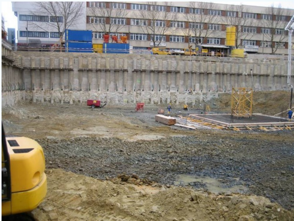
View after reaching max. excavation depth
